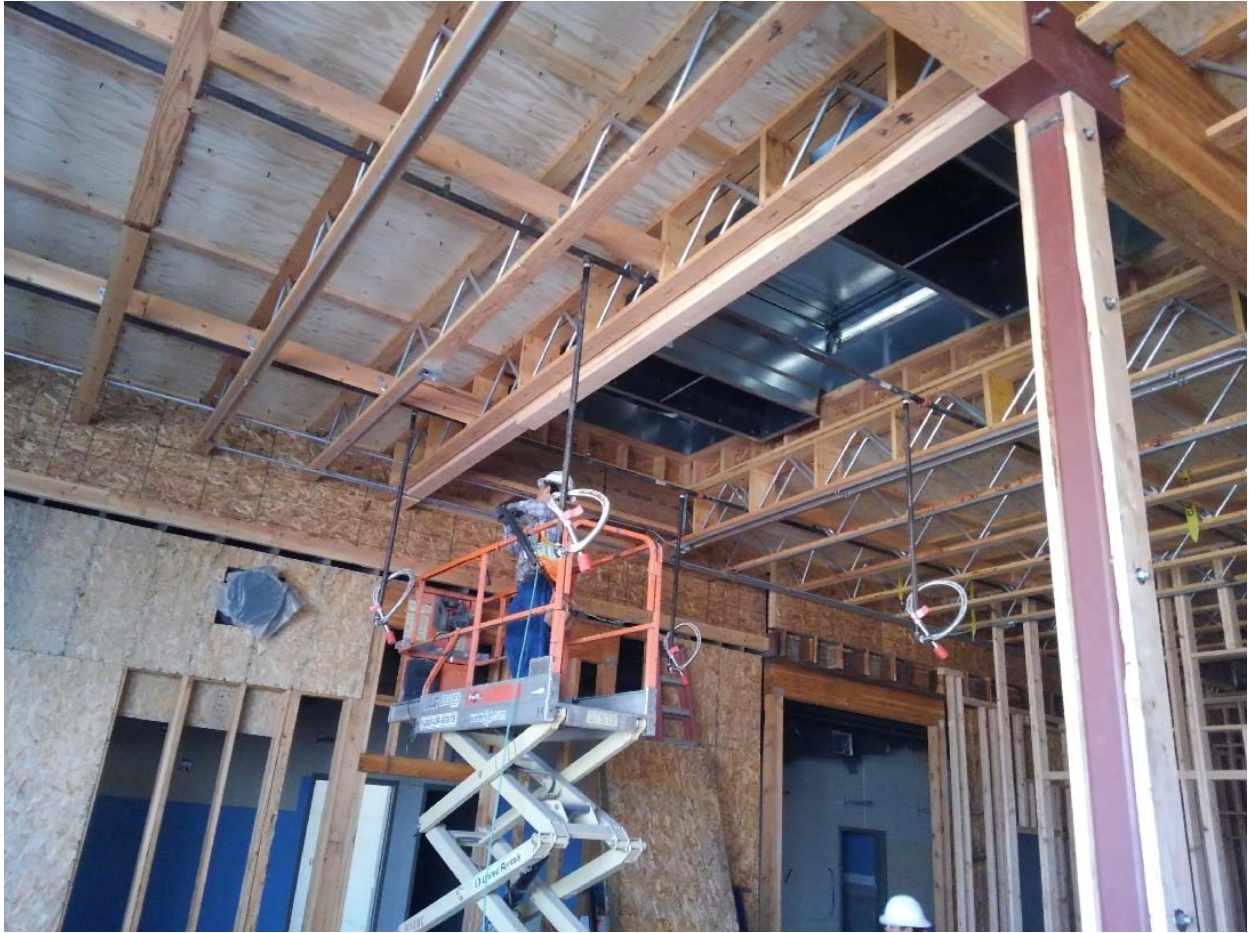
Framing on the third floor (new construction portion) is about 75% complete.
