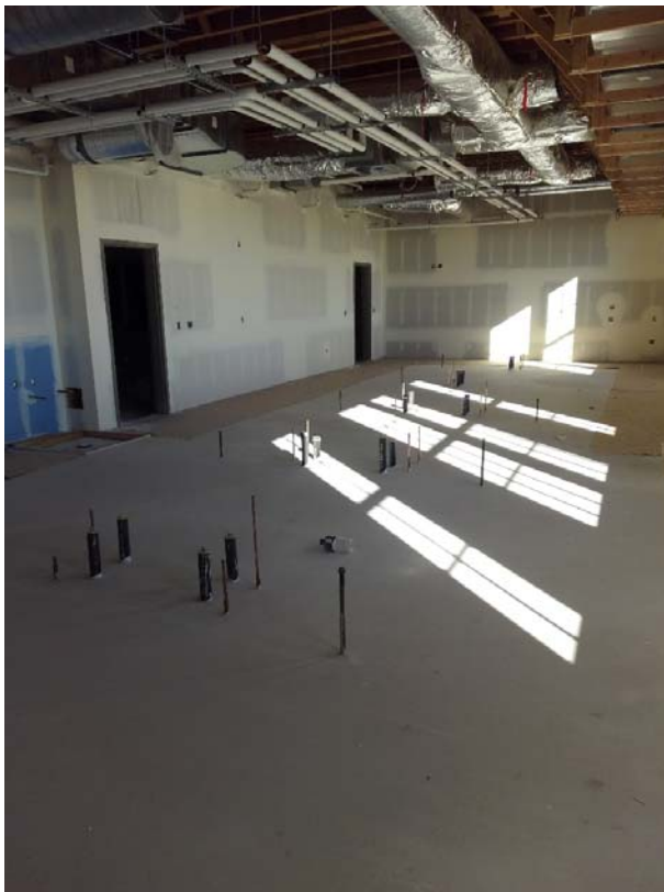
The Chem. room...ready to get a first coat of paint.
