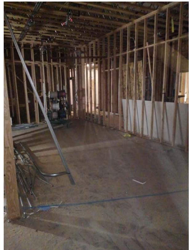
The staff lounge/work area sans sheet rock.
