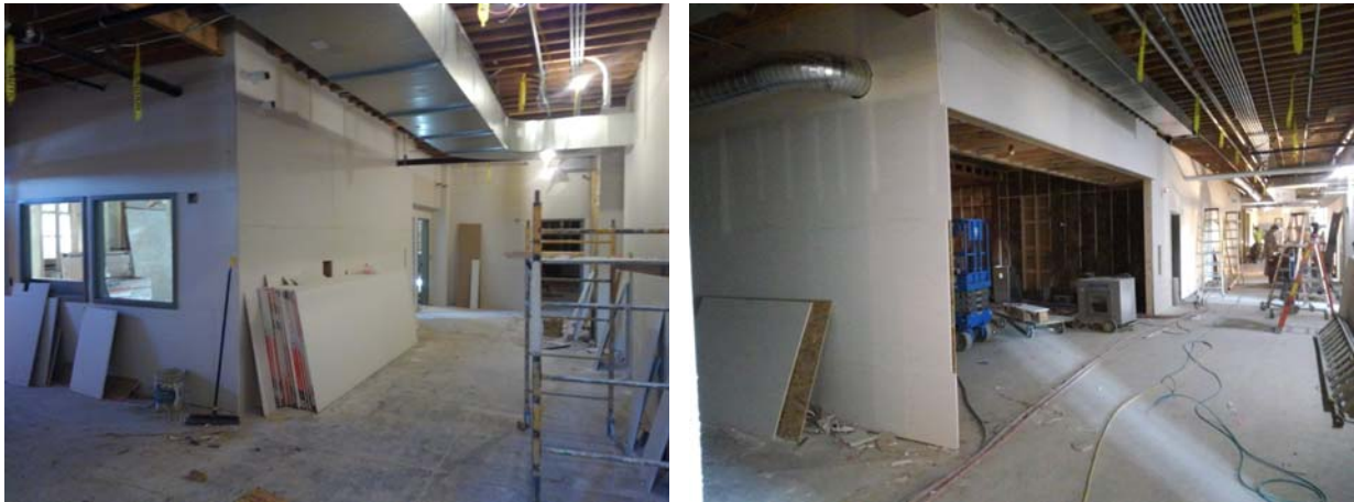
1 st floor hallways looking like...well, hallways!
