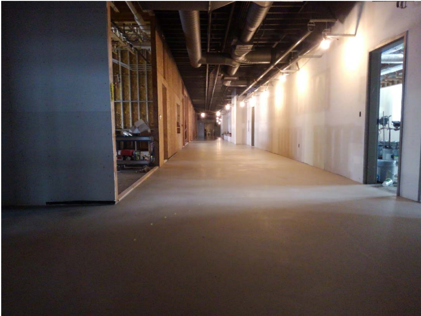
The Third floor hallway, looking towards Pel Court.
