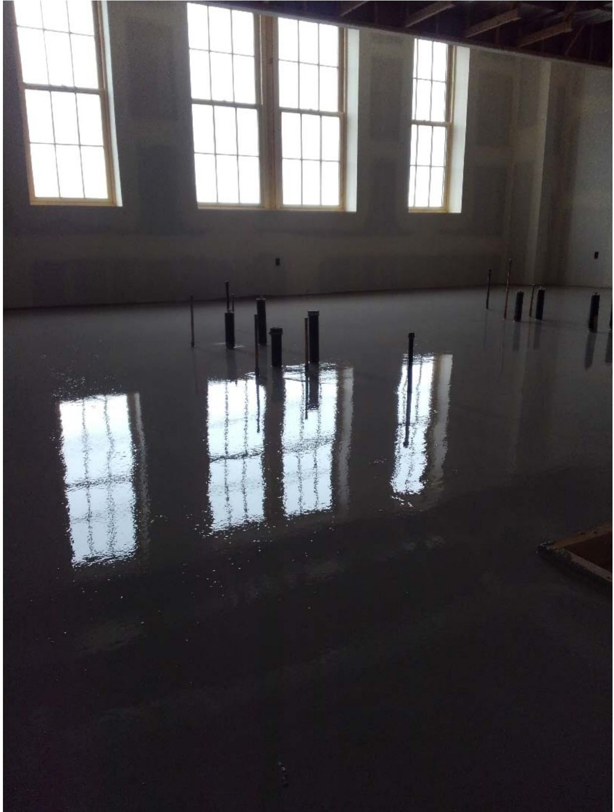
The completed Chemistry room in the curing process.
