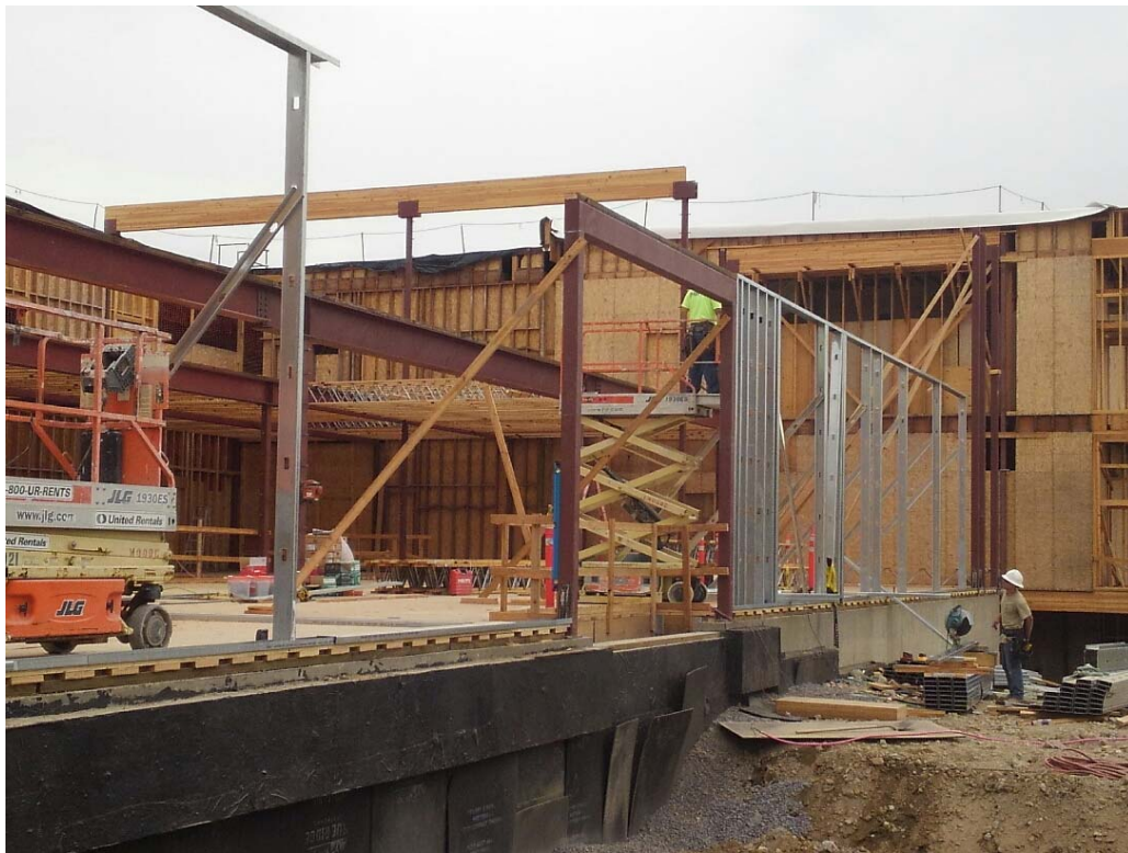
Construction is underway on the Monclaire Street North Wall!!
