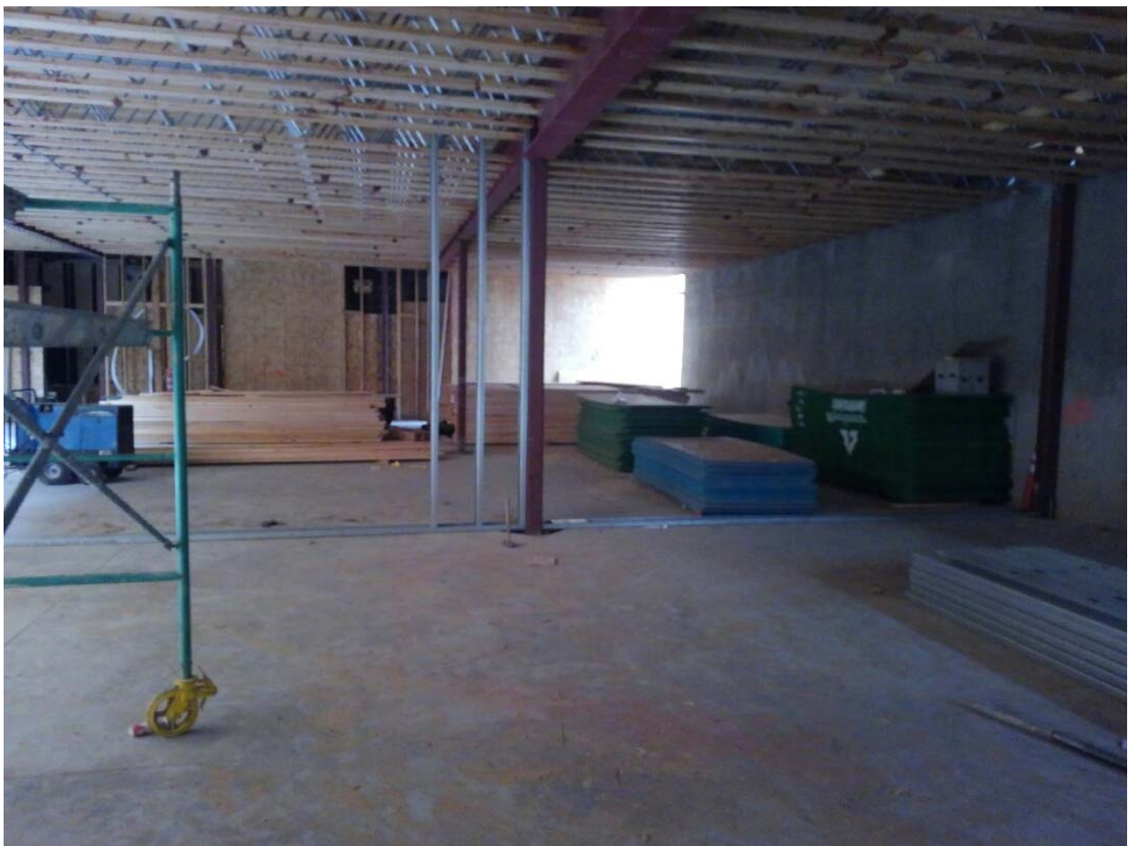
The First Floor is completely covered over.
