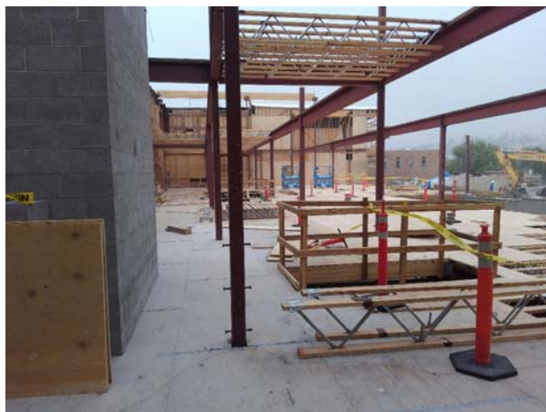
Second floor joists and the sub-floor sheathing are nearly complete... Third Floor well under way!
